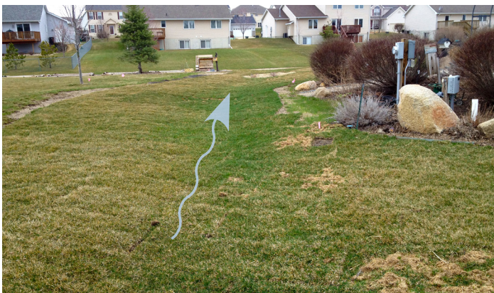
Most people would not realize that a stormwater practice is installed at this site. This Cedar Falls backyard bioswale will ensure a dry, mowable, and usable water management area. Permeable soil, a perforated subdrain and subtle earthen berms help infiltrate most runoff. Mow turf grass as high as possible to maximize vegetative cover.
