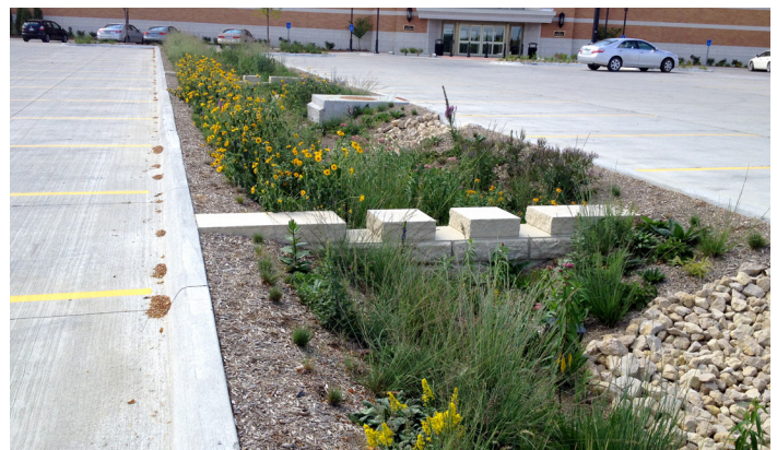
Stormwater runs off large parking lots very quickly. Bioswales are a great way to capture and infiltrate runoff from small events. Large events are conveyed to a storm sewer intake at the bottom of this swale. This bioswale provides an aesthetically pleasing green space in this Coralville parking lot.
