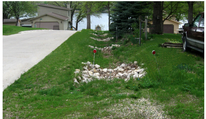
A newly completed bioswale with rock checks in a road ditch above East Okoboji Lake reduces runoff and sediment that used to be delivered to the lake with each runoff event. Rock checks help hold and infiltrate stormwater.
