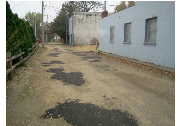
Before photo of alleyway in Clinton
