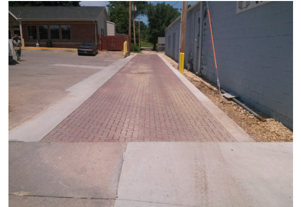
Completed permeable paver alleyway in Clinton
