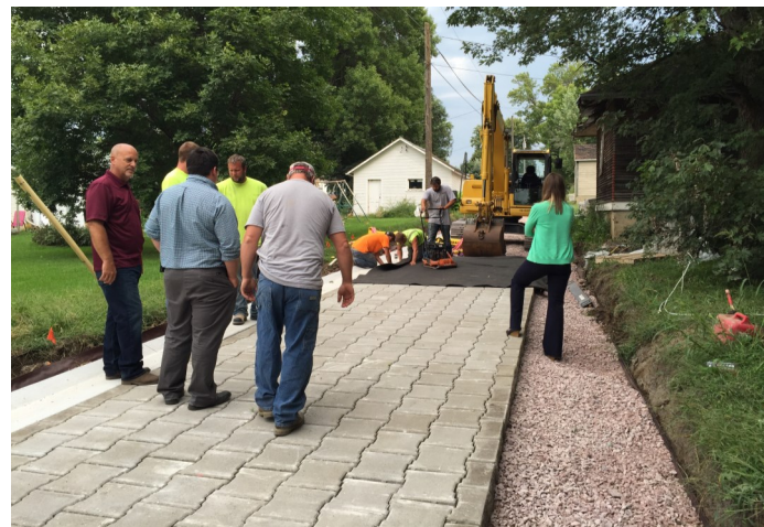
Permeable paver alley being installed in Kingsley
