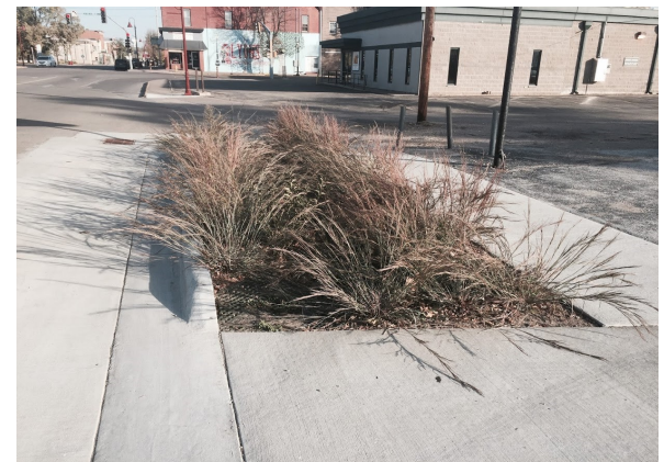
Bioretention cell manages street runoff in Clinton
