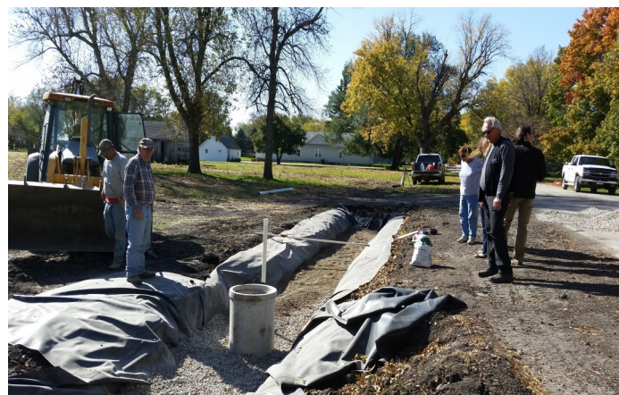
Bioretention cell being installed in Lohrville
