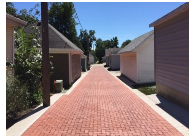
Permeable paver alley in Cedar Falls
