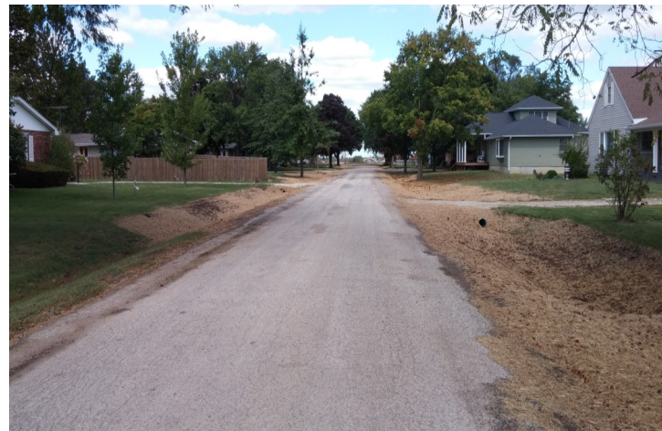
Bioretention cells alongside roadways in Donnellson
