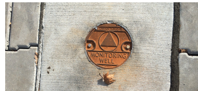
Monitoring well for water quality data collection.
