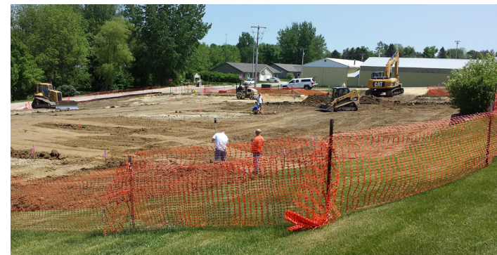
Site grading for the permeable paver parking lot.
