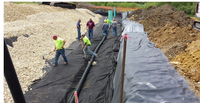
Installing the perforated subdrain in the rock base below the pavers.
