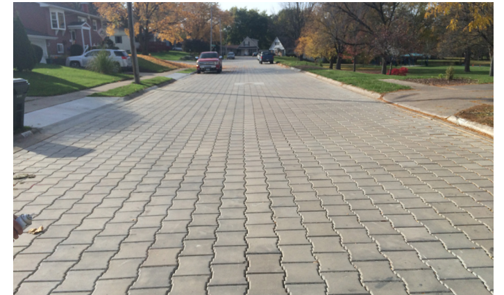
Completed installation of Dover Court in Davenport.
