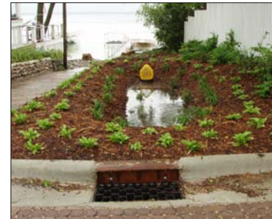
Permeable pavers and a rain garden protect Clear Lake from polluted runoff. Runoff is temporarily impounded and infiltrated to remove pollutants that otherwise would flow directly into the lake.
