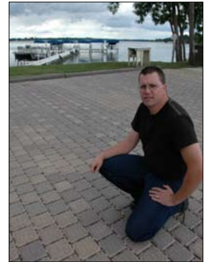
Pervious paving at Triggs Bay Resort eliminates polluted runoff and protects East Okoboji Lake.
