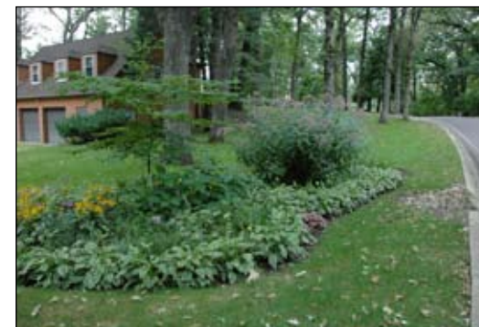
Runoff enters a rain garden thru a curb cut on Lakeshore Dr in Okoboji. Rain gardens treat and slowly release dirty street runoff.
