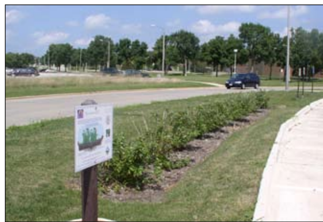
A rain garden catches runoff from a new parking lot on the campus of UNI, as part of the Dry Run Creek Watershed Project. UNI has installed multiple practices to reduce runoff and protect water quality.
