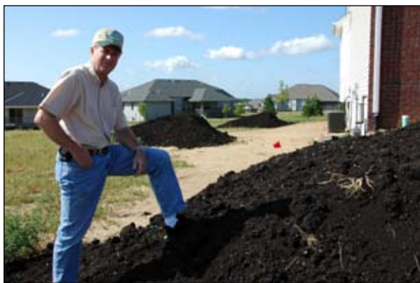
Rich oversees soil quality restoration at a newly constructed home. Construction causes soil compaction. Compacted soils increase runoff. This compost will be incorporated to increase organic matter content and soil porosity. Restored soil absorbs more rain, sheds less runoff, and requires less fertilization and irrigation.
