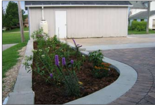
Woodard Insurance and Realty – a main street business in West Union – installed permeable pavers, a rain garden and a rain barrel to capture and treat roof runoff in the back of the building. This project serves as a model for the major "green street" revitalization project West Union is planning for the business district.
