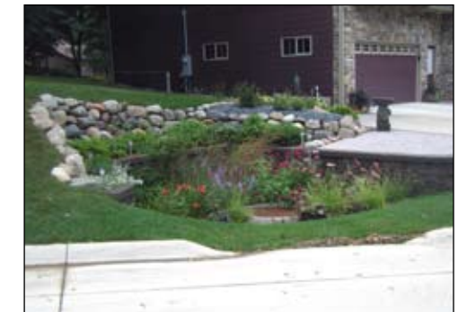
This rain gardens is one of fifteen installed to treat runoff as part of Iowa's first "green street" project in Okoboji.
