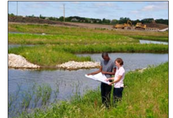
These constructed wetlands treat storm water from a residential subdivision in Prairie Trail before it's released into the stream.
