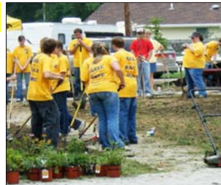
West Pottawatomie SWCD partnered with Habitat for Humanity and a church youth group to install rain gardens and restore soil quality at a new home in Council Bluffs.
